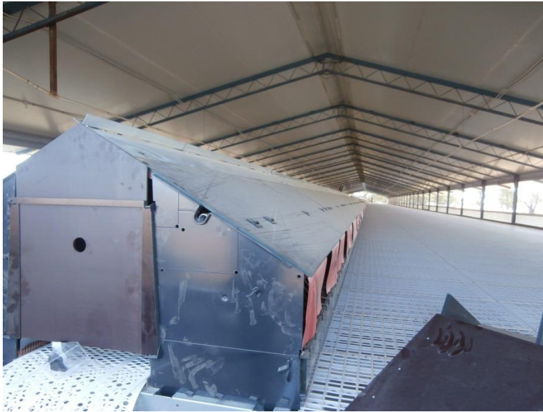
Photo 3.1 Shed Fitout for Free Range Layers
